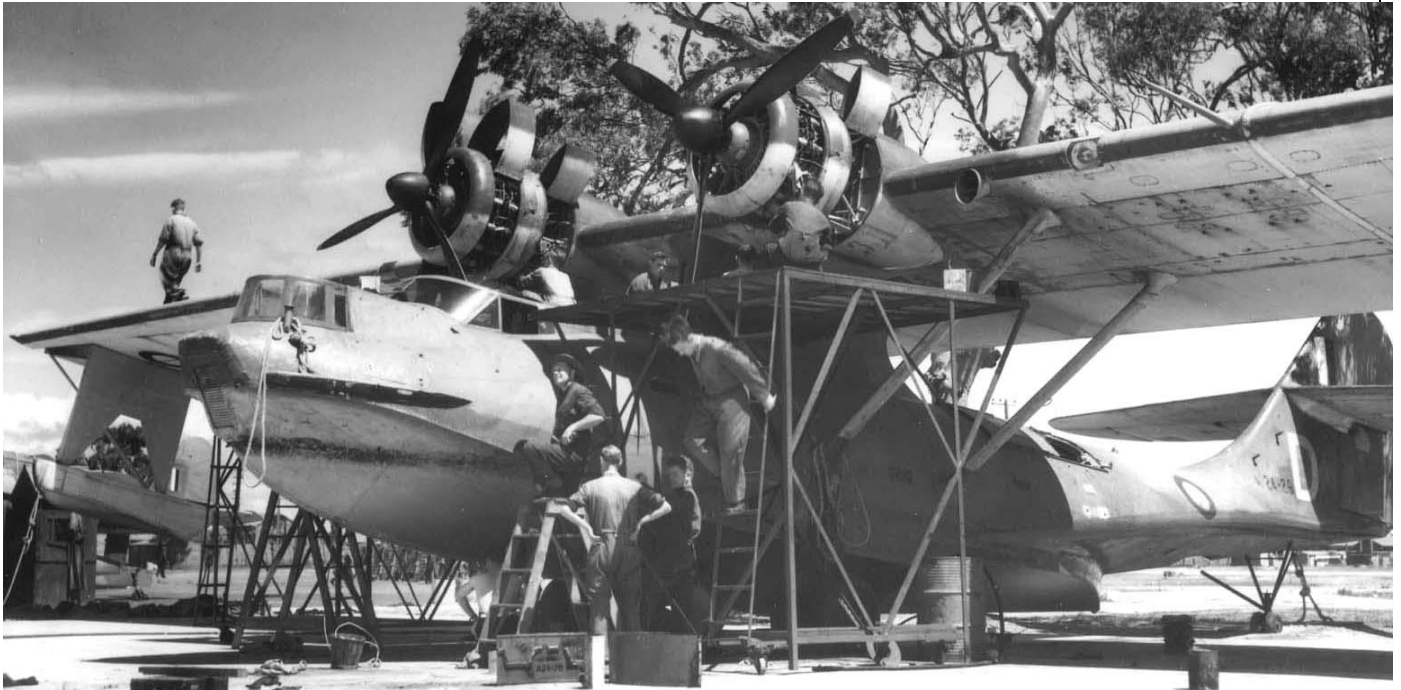
The original configured PBY-4 with propeller spinners, rounded rudder and no blisters [RAAF]
