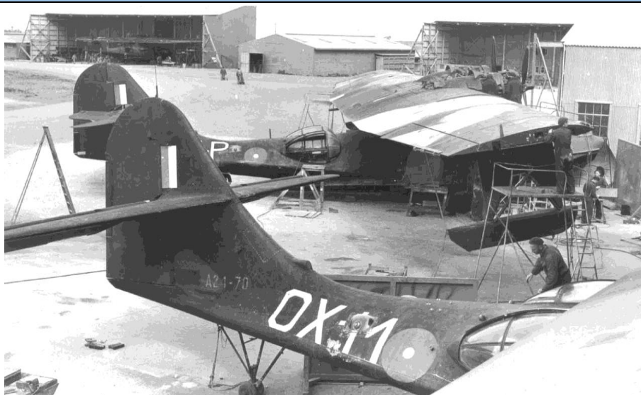
A24-70 OX-M with 11SQN A24-69 FJ-P at 1FBRD Lake Boga for PBY-5A(M) modification AUG 1944
